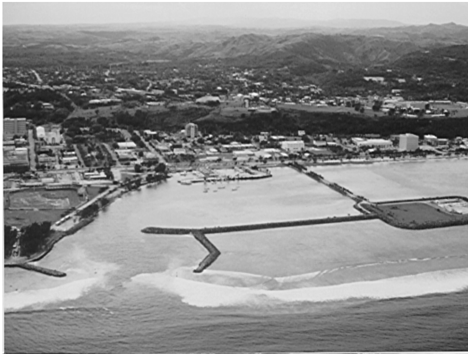
Figure V-5-35. Breakwaters protecting small boat harbor from waves and wave-generated crosscurrents on reef, Agana, territory of Guam (May 1978)
