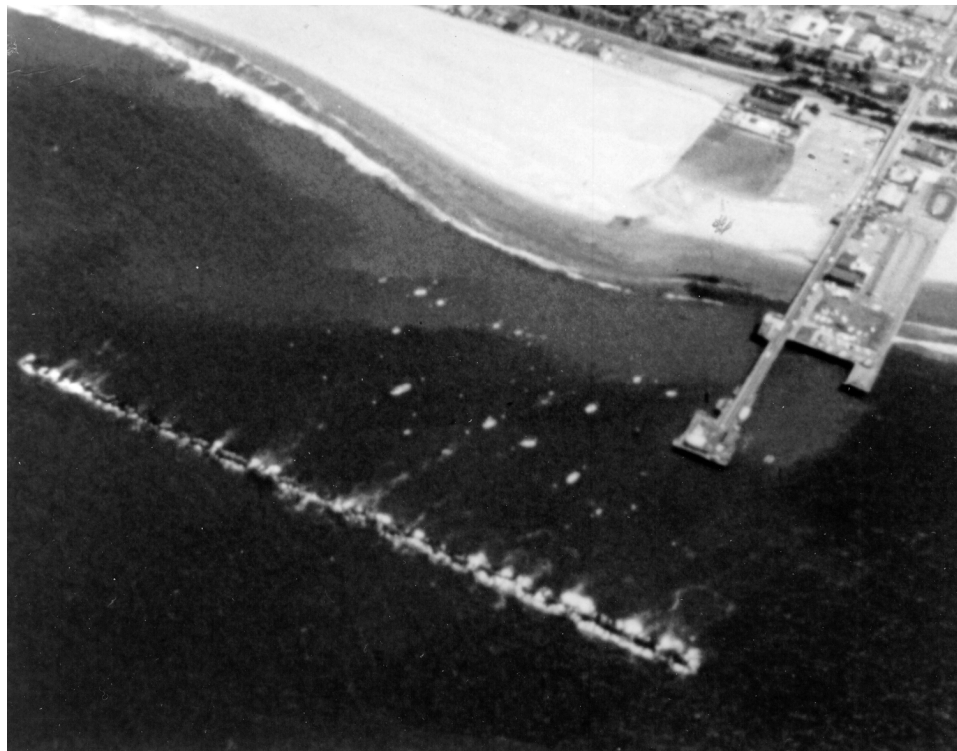
b. Deteriorated breakwater allowing wave transmission
